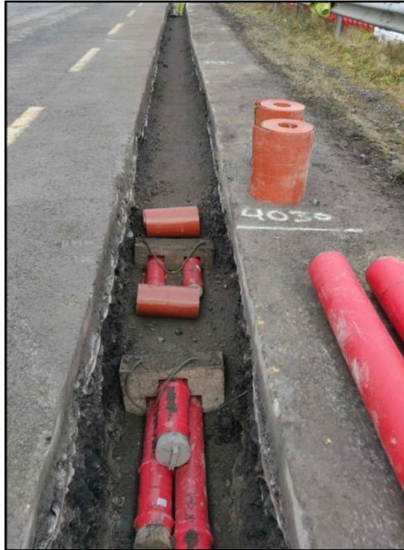
Plate 2-1 110Kv Cable Trench View
