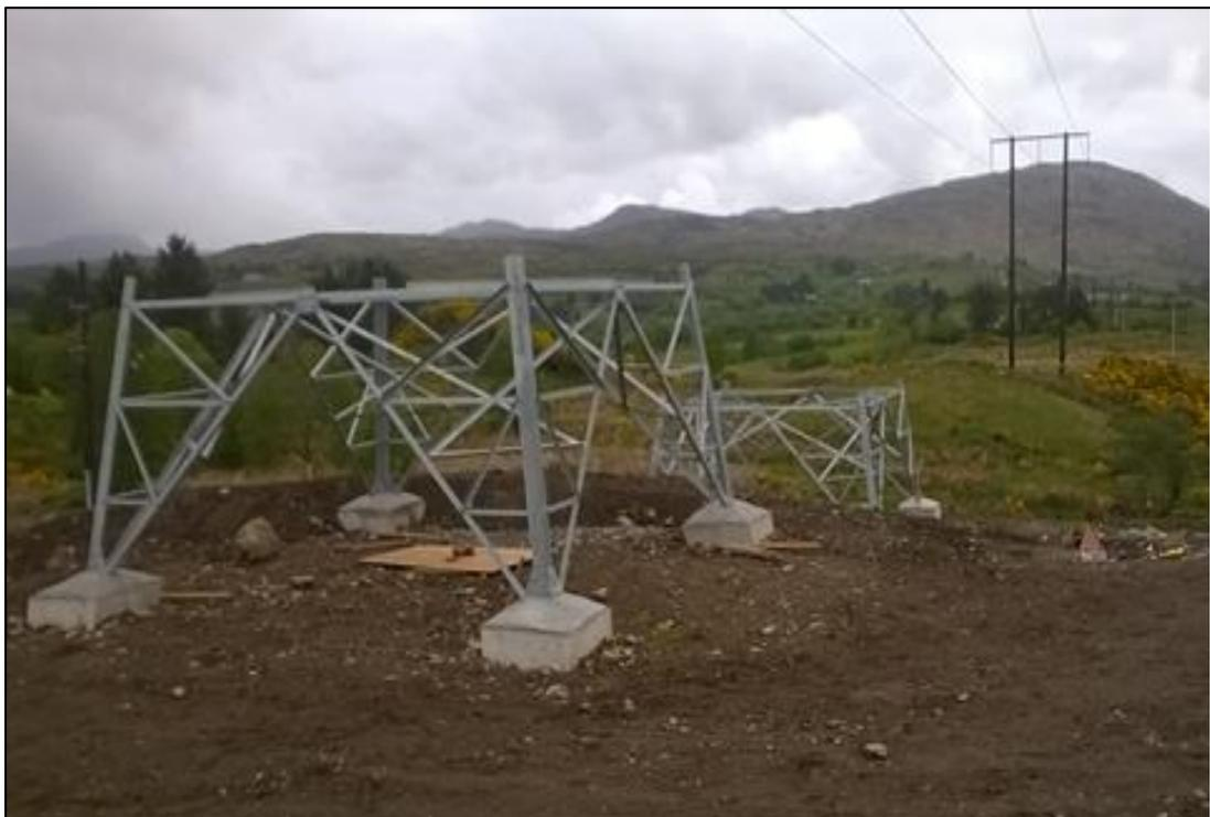
Plate 2-3 Steel lattice tower foundation complete (example image)
