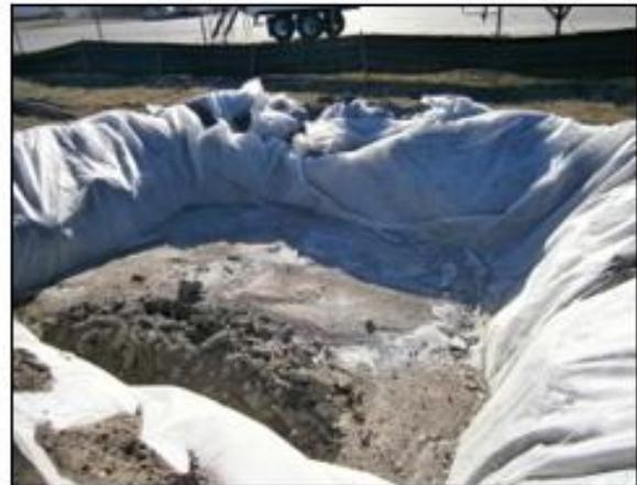
Plate 3-1 Typical concrete wash out areas
